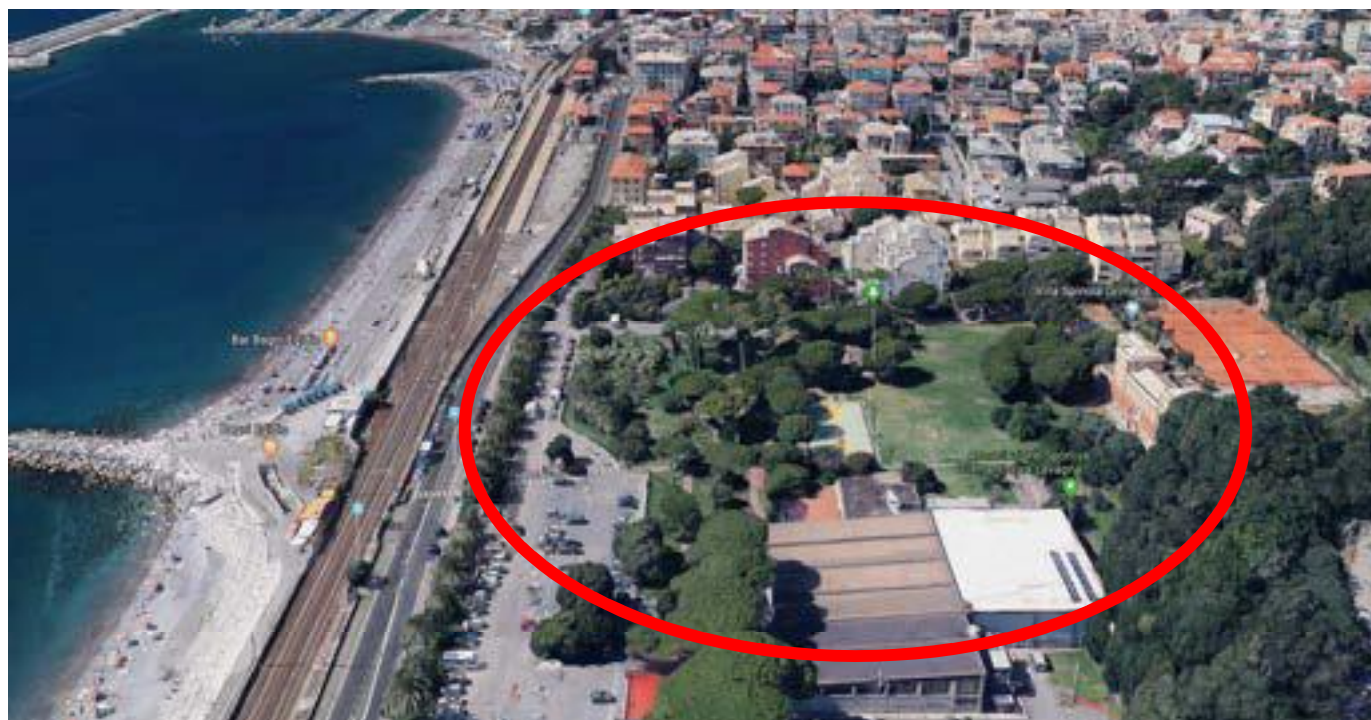
Framing park Villa Grimaldi Spinola in Lavagna (GE) site of the pilot action of "sustainable urban space"
